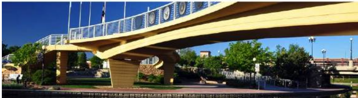
Veterans Bridge - Historic Arkansas Riverwalk, Pueblo
