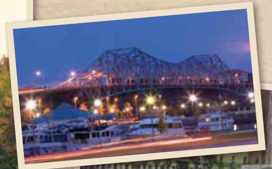
Florence Bridge, AL
